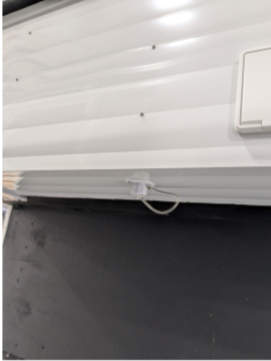
Water Drain Outlet
