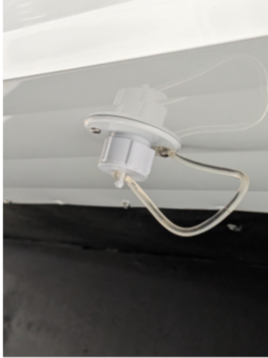
Water Drain Outlet (close up)
