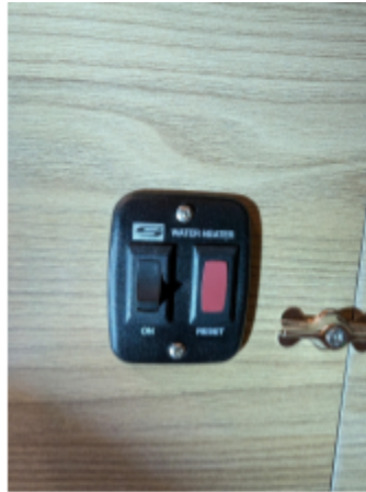
Water Heater Switch
